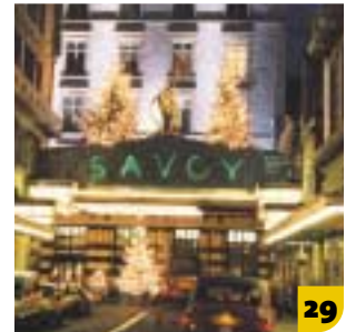
New Lease on Old Wires
